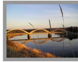
Nicholsville Bridge Photo Compliments of Dr. Greg Wood
